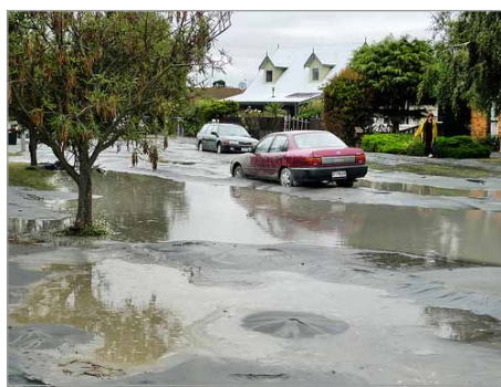
Sink holes and liquefaction on roads, Avonside in Christchurch
