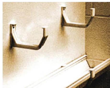
Plastic brackets to support rain guttering
